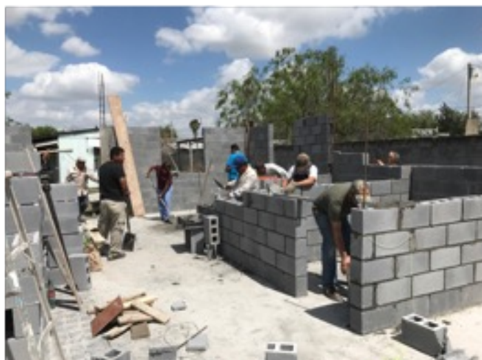
The River City New Braunfels group built the block walls
