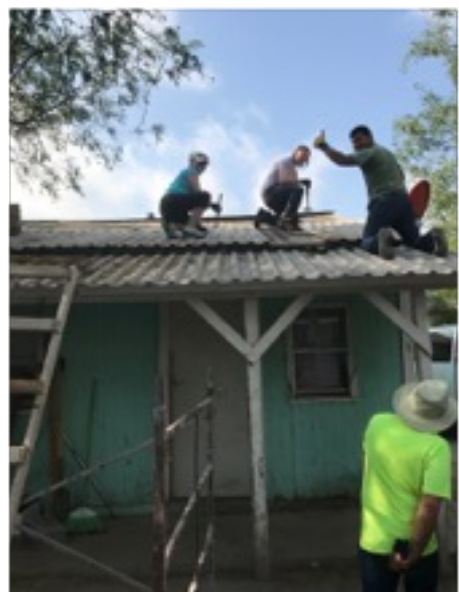
Epic Church from Baltimore removed the trusses from the old house.
