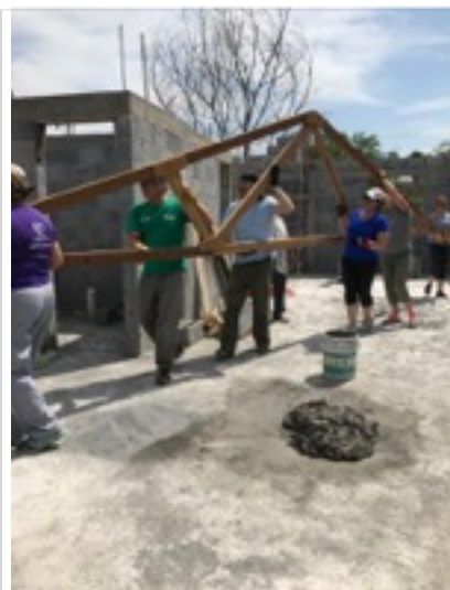
The old trusses were moved to the new house
