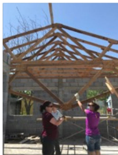
And lifted in place
