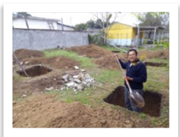
Pastor Antonio works on the foundation for his new home.
