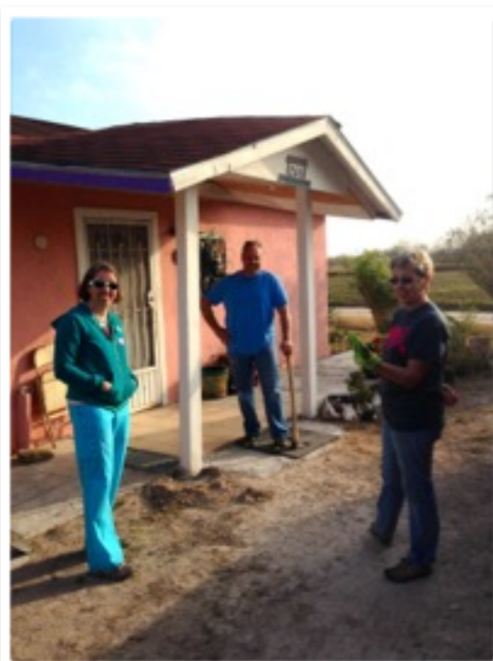
Folks from Anna repair the roof on Olga Berman's porch.
