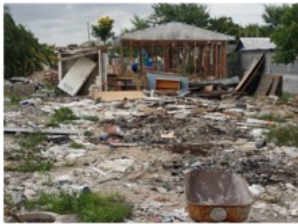
Demolition in progress on the lot next to the Pastor's house.
