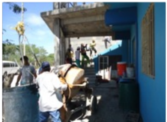
Then it's carried to the second floor in 5 gallon buckets
