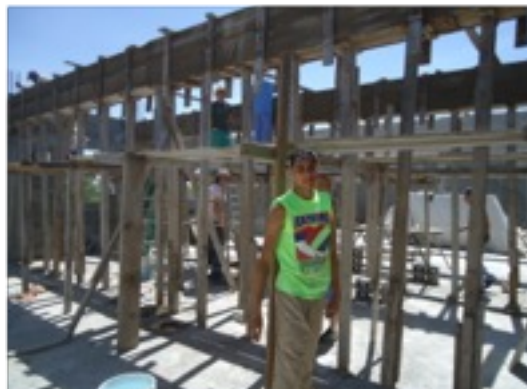
Grandson, Isaiah, is on the second floor work crew.
