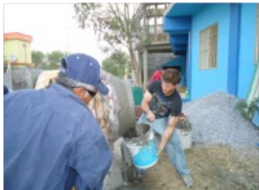
Grandson Brandon fills buckets with concrete
