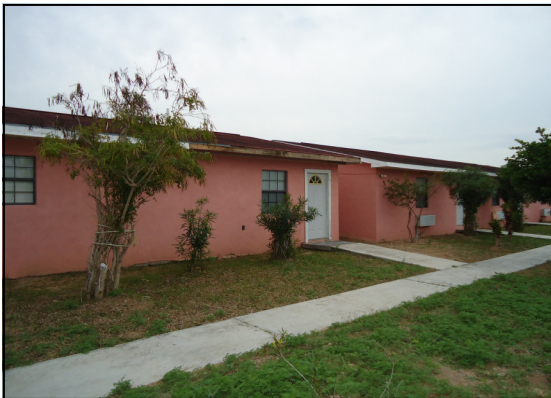
Missing fascia and soffit
